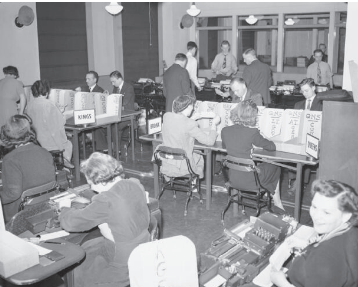
Tabulators record the Associated Press election returns in the offices of IBM in New York City on Election Day, Nov. 3, 1942. The returns are received on the teletype machines (background) and recorded with the aid of the numeric punching and printing machines in the foreground. (AP Photo/Matty Zimmerman)
